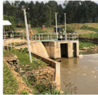
Intake: majority of water is temporarily diverted into the channel
