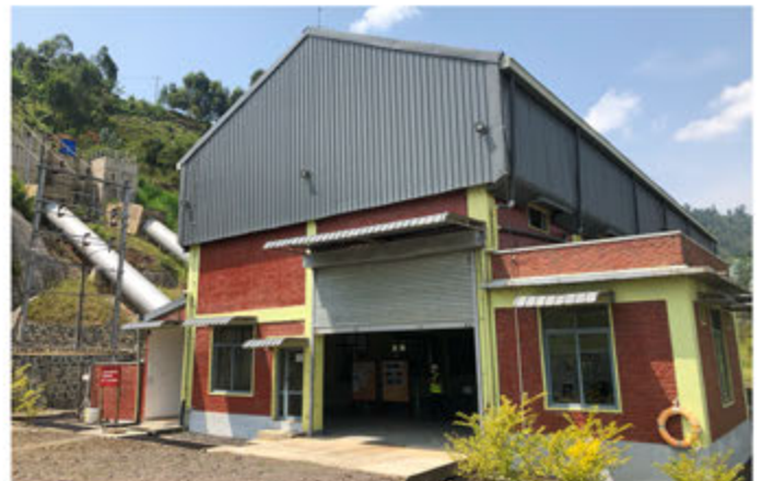
Penstock and Powerhouse: end of channel water is gravity fed into the powerhouse
