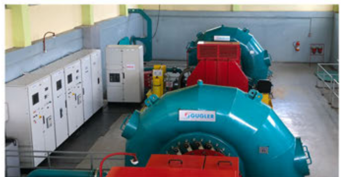
Turbines: movement of water is converted to energy to be fed to the grid
