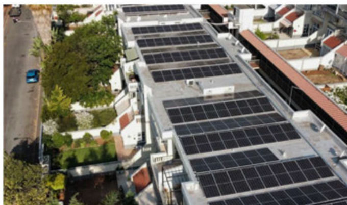
A new rooftop solar PV and battery storage system provides energy to tenants of a 54-unit apartment block in Johannesburg, South Africa
